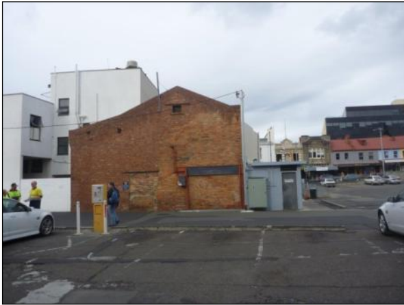
Figure 73: Rear end wall of 147 Elizabeth Street, constructed in c.1925 as a cool store.
