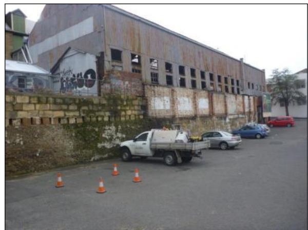
Figure 88: Sandstone, brick and rendered stone boundary wall separating the car park from 37-47 Melville Street.
