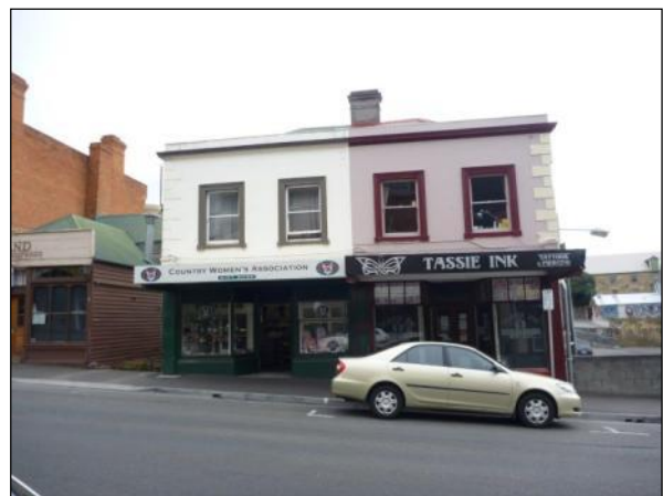
Figure 76: 163 (right) and 165 (left) Elizabeth Street.
