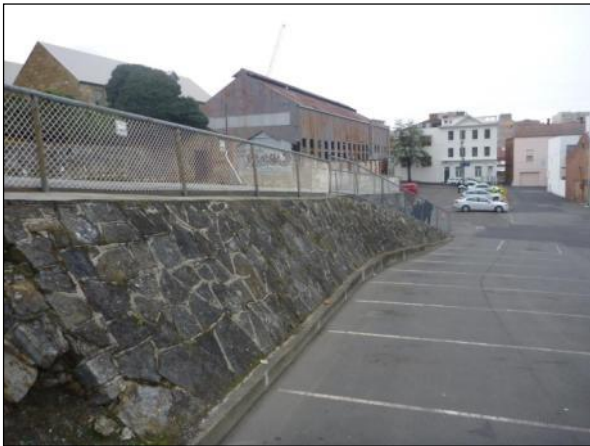
Figure 83: Bluestone retaining wall dividing the two Brisbane Street ends of the car park.
