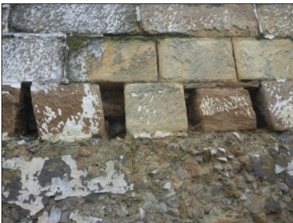
Figure 89: Slots in sandstone boundary wall to accommodate beams for former foundry buildings.
