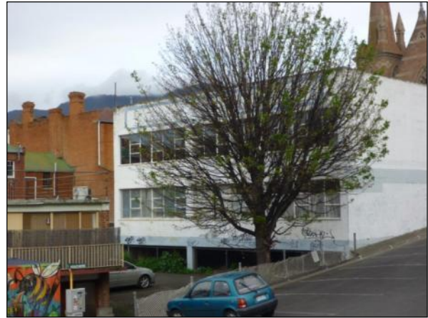
Figure 80: Southern elevation of 64 Brisbane Street.
