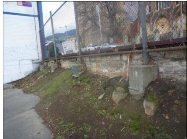
Figure 82: Sandstone retaining wall dividing the car park from the street.
