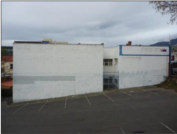
Figure 79: Eastern elevation of 64 Brisbane Street.
