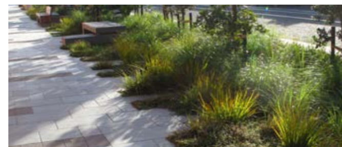
Image 30 Swales and rain-gardens as a part of streetscape WSUD
