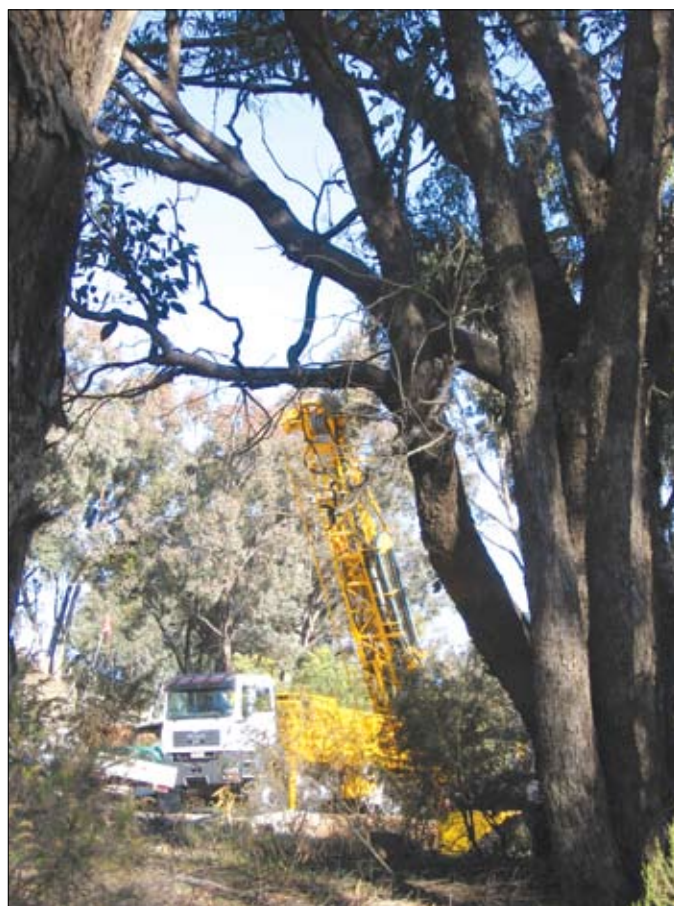
Drilling at Cadia East, NSW. Project P2.L1.
