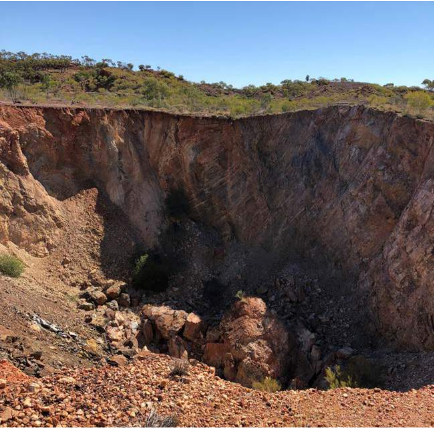
The Corbould collapse zone, Mt Elliot IOCG deposit, which was studied in the 'Mineral geochemistry vectoring' project. After mine closure, an area of structural weakness at depth propagated to the surface, resulting in the exposed void. Note the steeply dipping bedding in the far wall of the pit.
